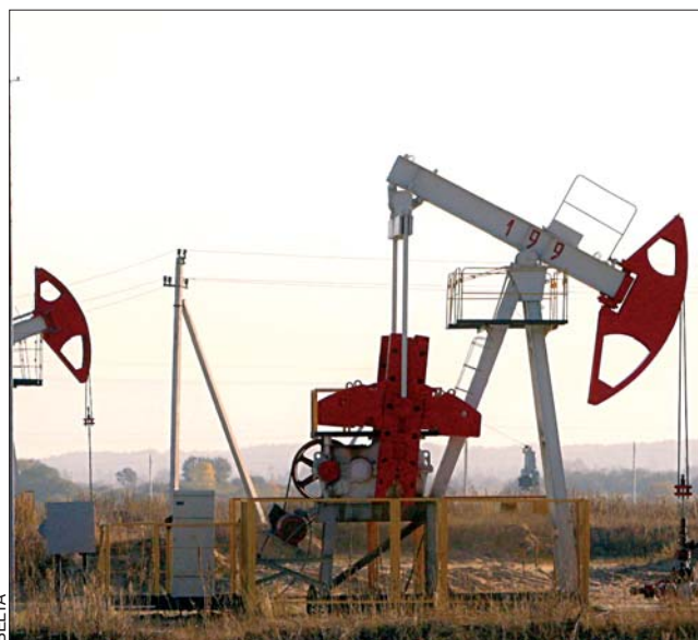
Oil pumps raise oil from below
