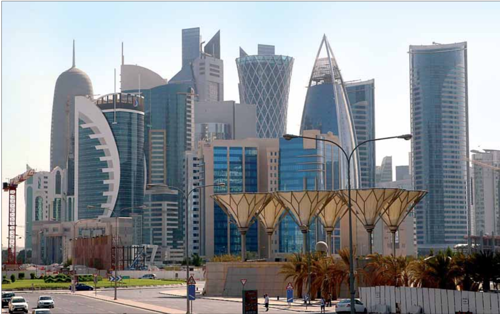
Qatar's capital of Doha vividly demonstrates rapid state development
