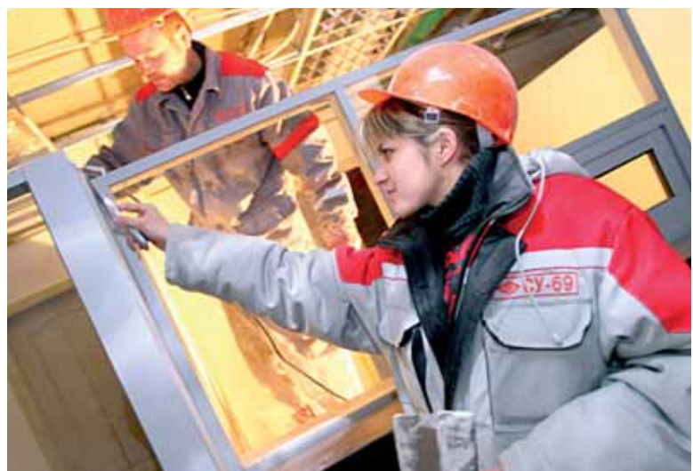
Specialists involved in final finishing works
