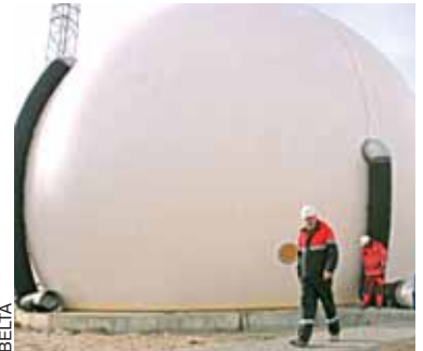
First biogas generated in Brest
