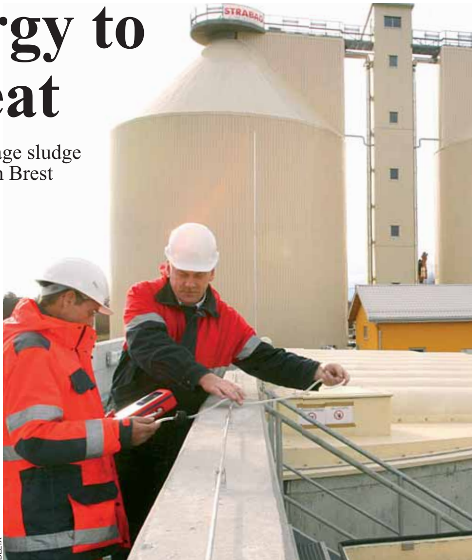
Specialists from Brest's Recycling Plant measure gas levels
