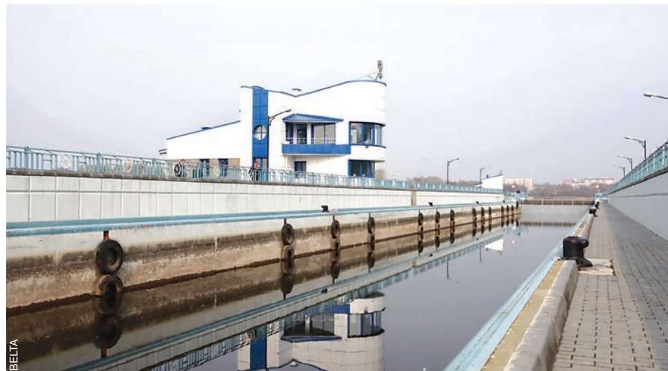
One of infrastructure objects of the Dnieper-Bug waterway
